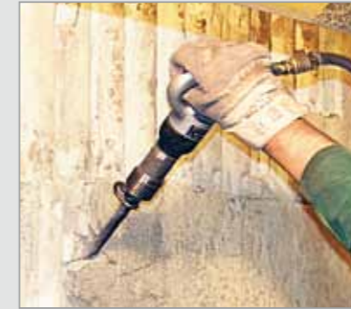
Effortless removal of plaster and tiles
