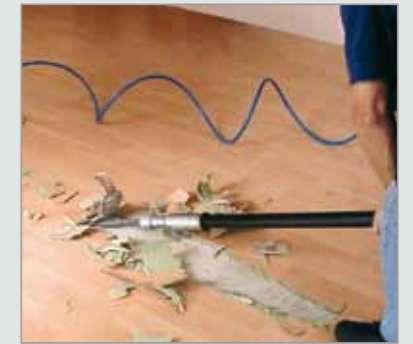
Floor coverings stripped with ease
